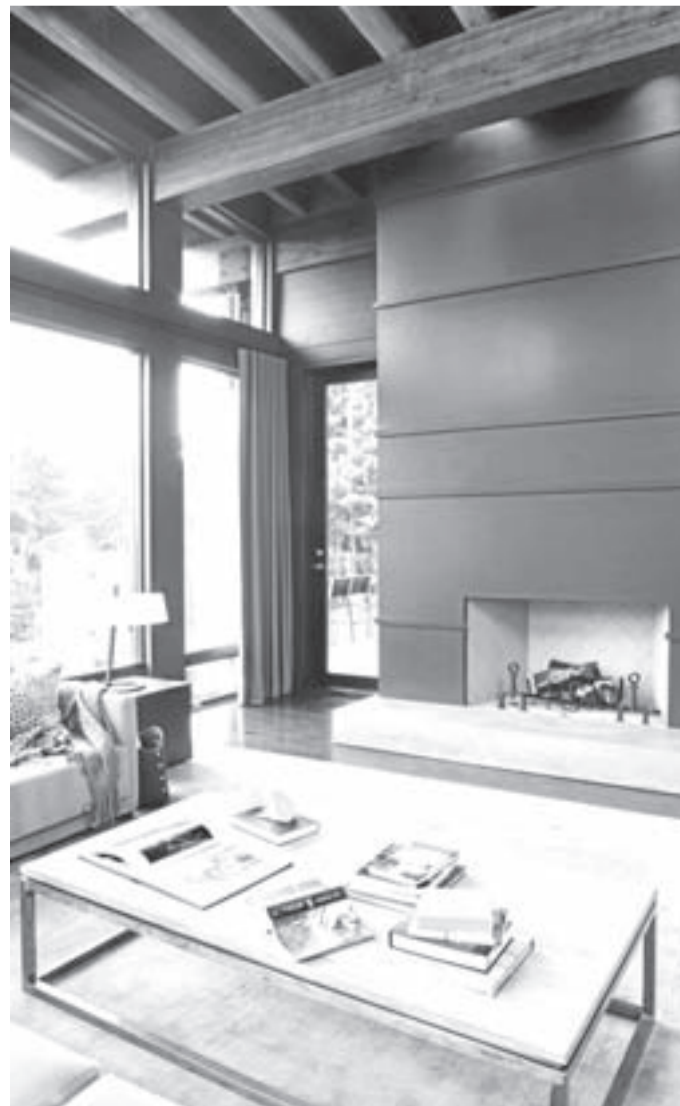
In the great room, the fireplace made of cold-rolled steel is attached with a special system of cleats that conceals the joinery. The 18-foot ceiling is finished with espresso-stained cedar beams. BARRY CALHOUN
